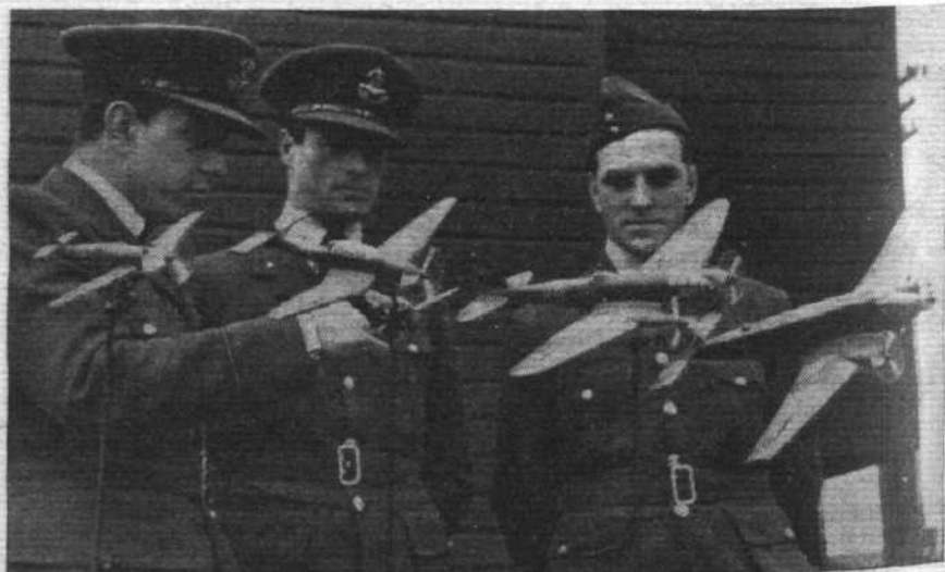
Scale models of German aircraft are used for instruction in zones of fire. Gun positions are represented by small illuminated bulbs.
